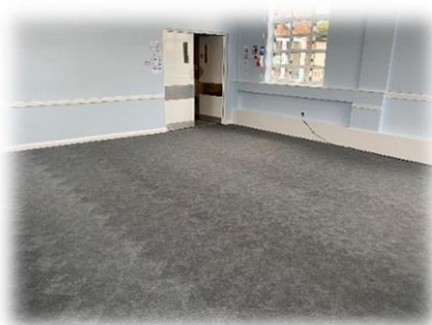
Meeting Room Refurbishment
