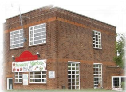
The Old Fire Station
